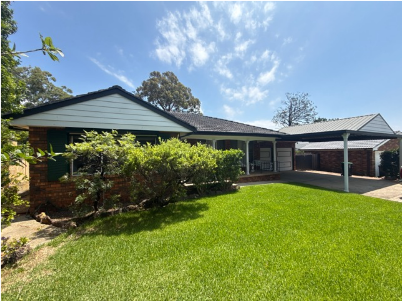
76 ROSINA CRESCENT KINGS LANGLEY
